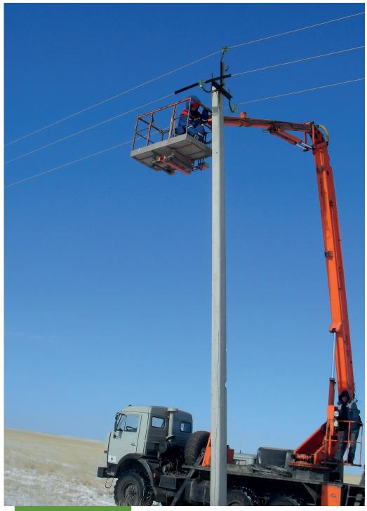
Fig. 1. In 2016 33 km of power lines were equipped by birds' protection devices
